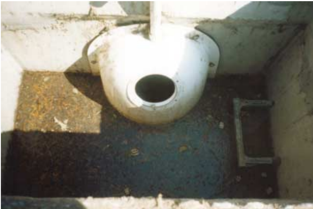
18 F SNOUT is shown with the access port open in a 2' x 4' inlet structure with a 15" CMP outlet and 4' of sump below pipe invert. This unit functions as an oil-water-debris separator trapping floatable debris, trash, oil and grease, and sediment.
