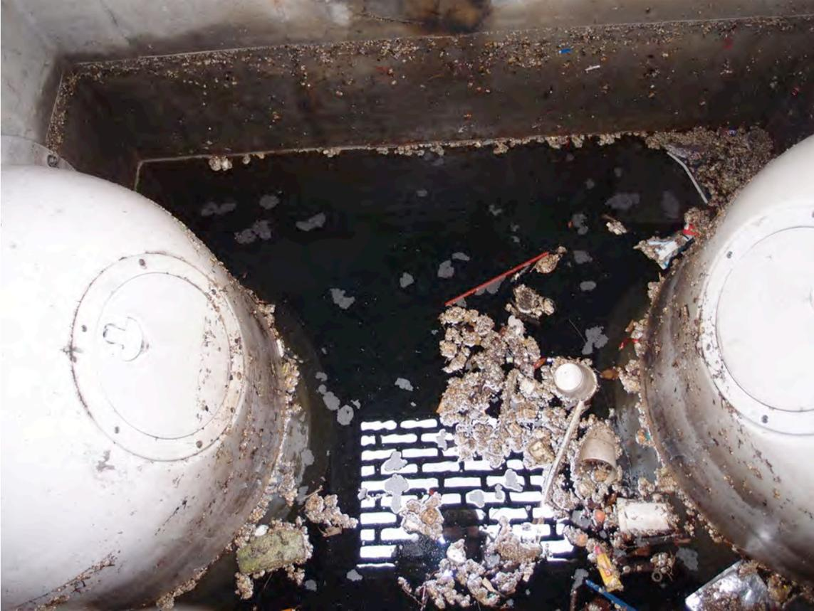
Figure 7, Near 3<sup>rd</sup> Avenue S., and Ocean Boulevard. Shown is a pair of 30F SNOUTs covering 24” perforated pipe
